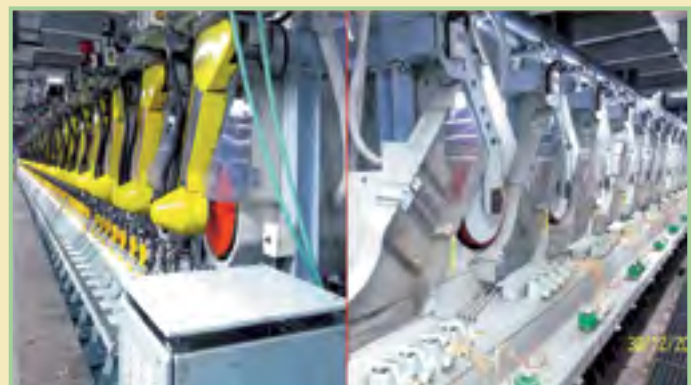
CAPACITY ADDITION TO CSY PLANT (MACHINES IMPORTED FROM CHINA)
